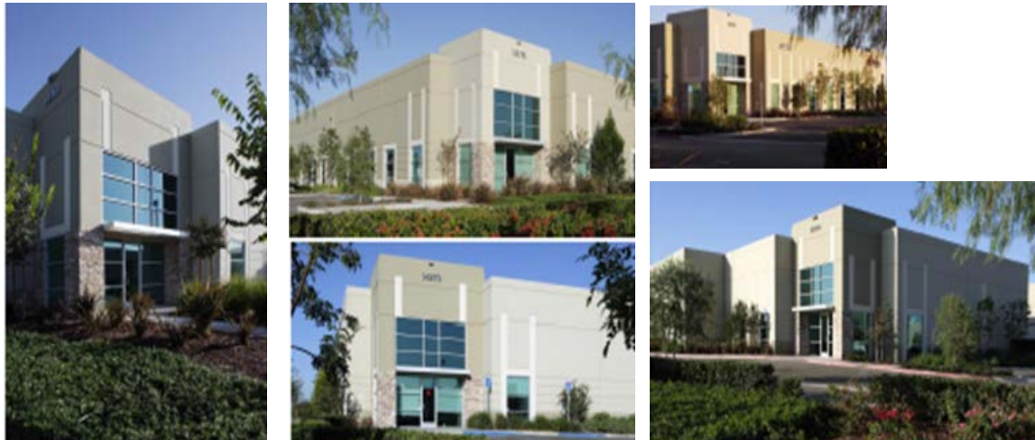
Examples of Light Industrial Buildings
