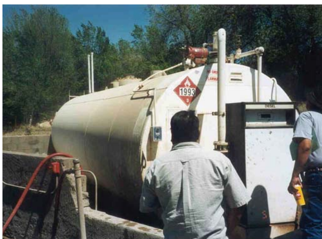
Upper left: Good example of secondary containment.
