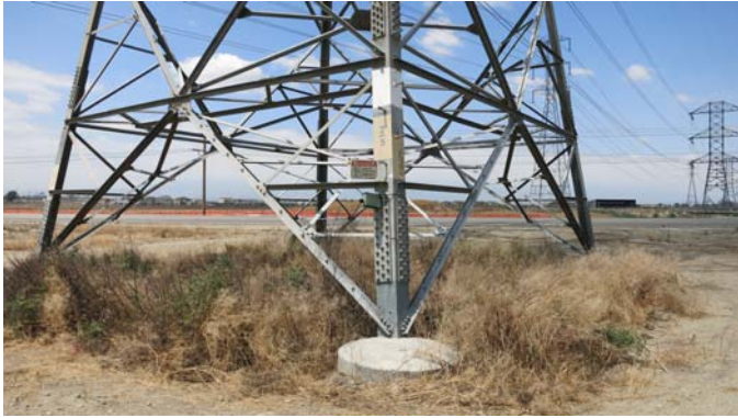
Noise Measurement Site A - looking north
