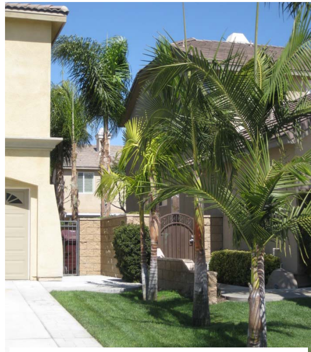
Return wall and gate between two houses
