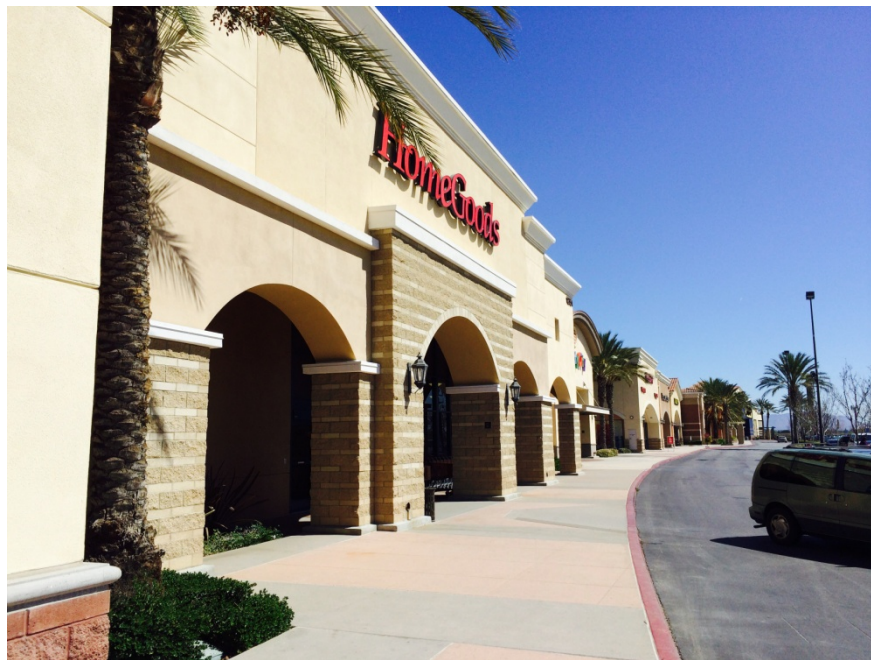
Use of arcades to visually link buildings
