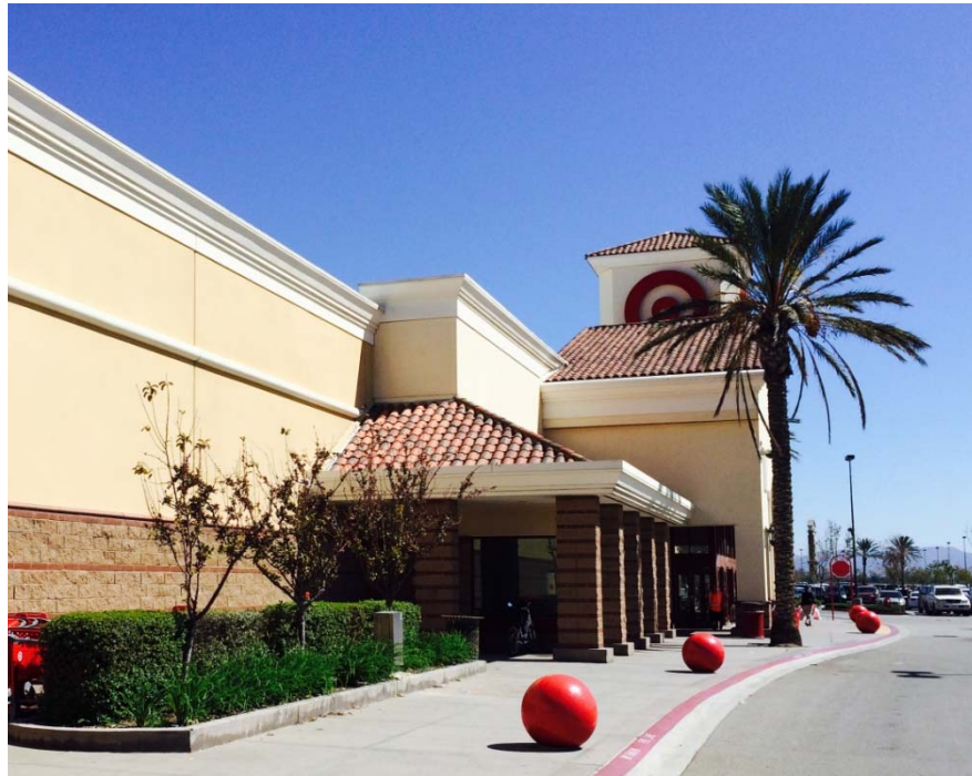
Example of well-articulated “big box” structure
