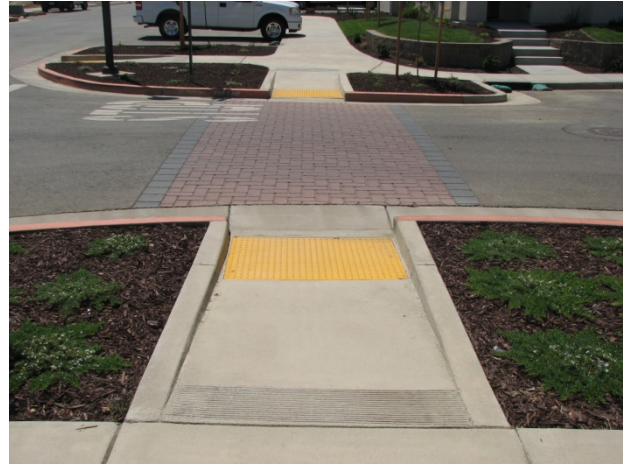
Enhanced paving defines the pedestrian crossing and adds visual interest
