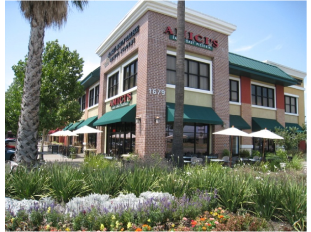
Buildings along street frontage
