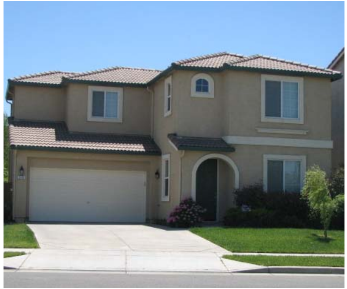
Roof articulation – hip roof
