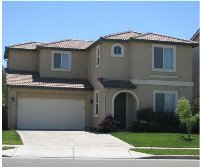
Roof articulation – hip roof
