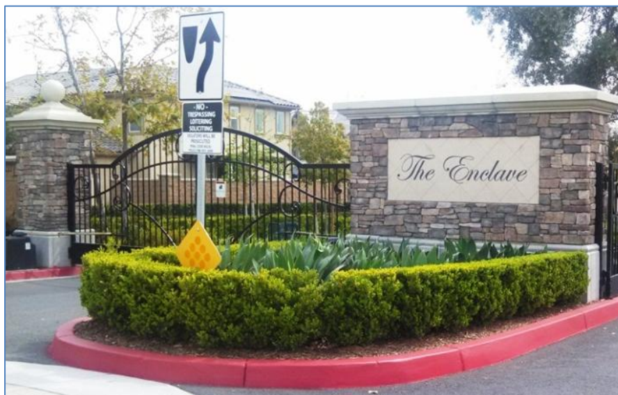
Example of attractive security gate
