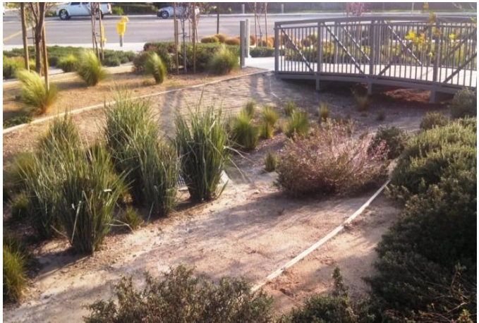
Water quality basin
