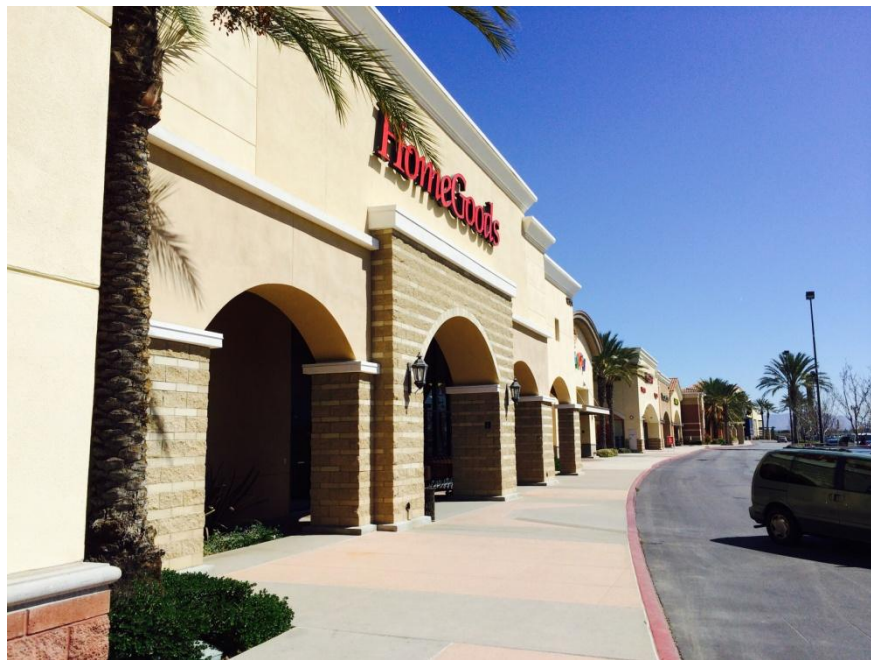
Use of arcades to visually link buildings
