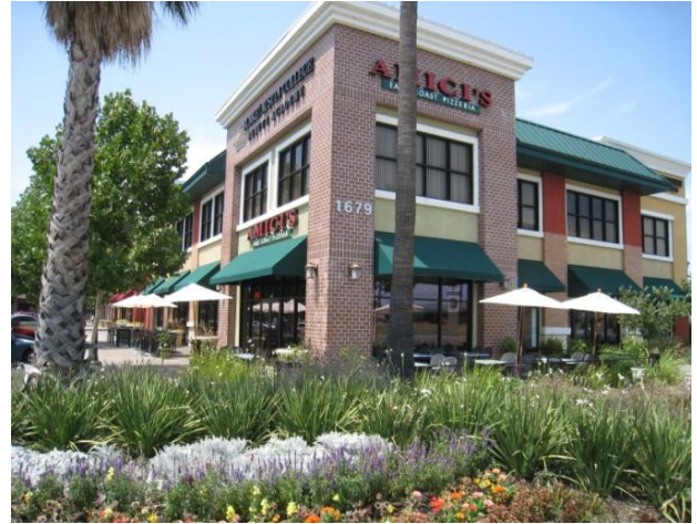
Buildings along street frontage
