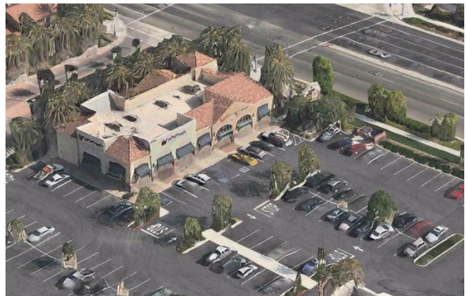
Parking lots on side of buildings
