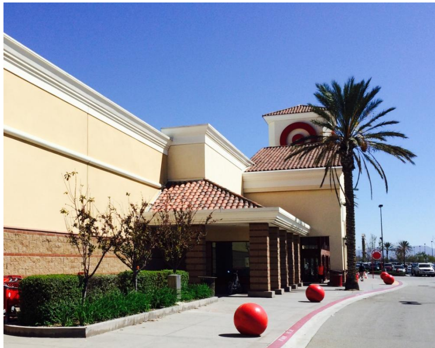
Example of well-articulated “big box” structure
