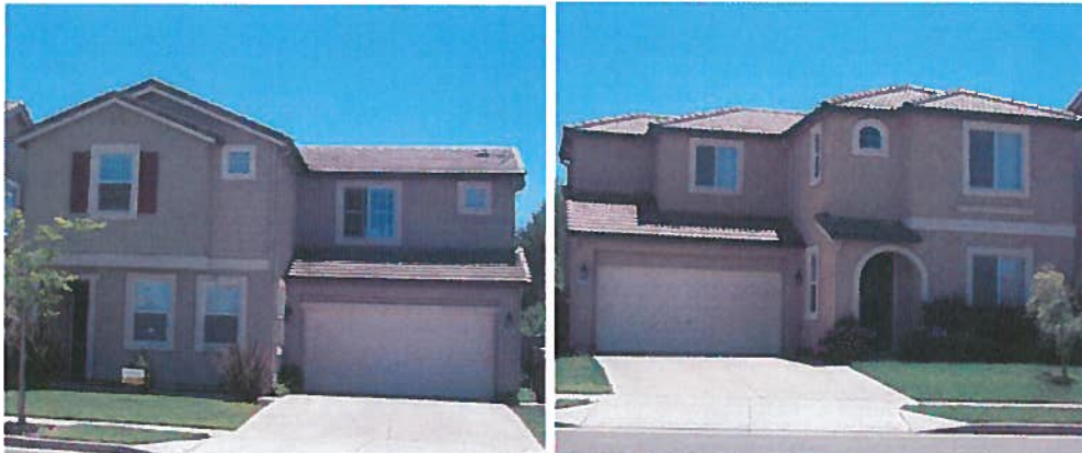
Roof articulation – gable roof
