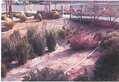
Water quality basin
