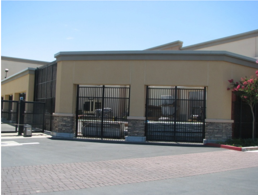
Screening of outdoor storage area
