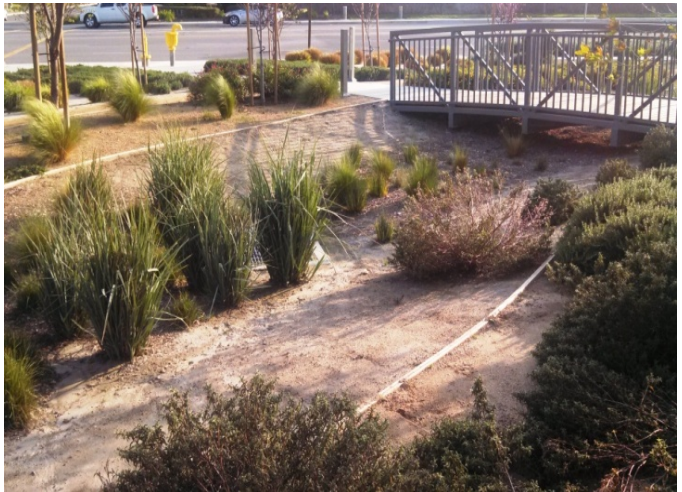
Water quality basin
