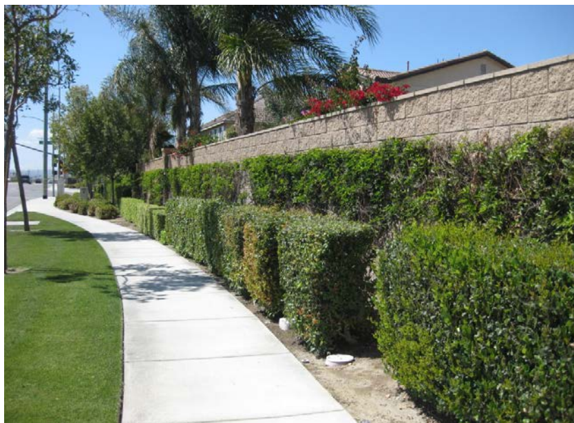
Use of vines and landscape to soften the appearance of walls
