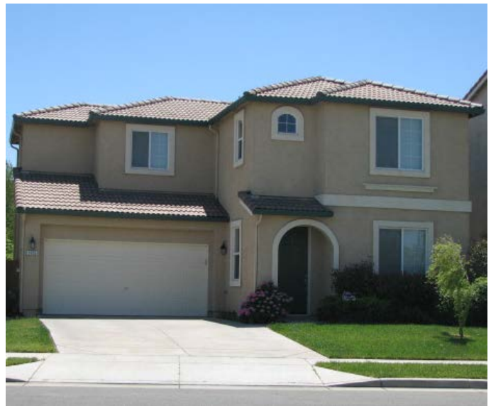
Roof articulation – hip roof
