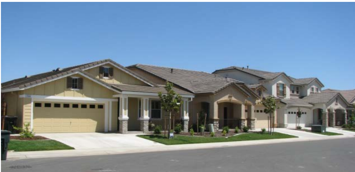
Three distinct elevations
