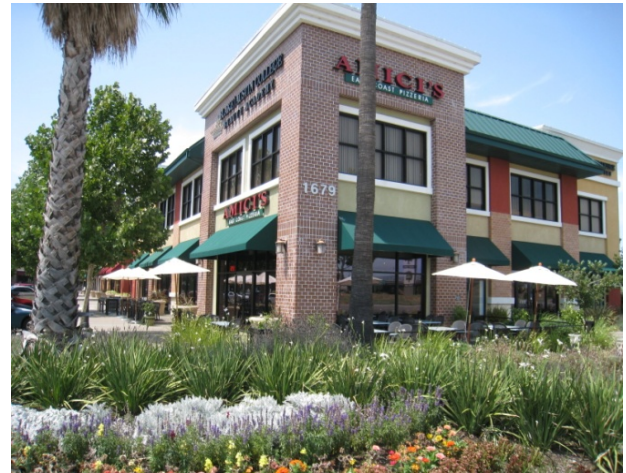
Buildings along street frontage
