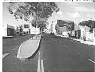
Provided engineering services for a project consisting of the rehabilitation of approximately 2.3 miles of Atlantic Avenue from Bixby Road to South Street in the City of Long Beach. The project included pavement reconstruction and rehabilitation, reconstruction of curb ramps per current ADA criteria, crossgutter and curb/gutter reconstruction, and signing and striping.
