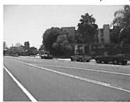
Provided engineering services for the rehabilitation of approximately 2,400 feet of Carson Street from Long Beach Boulevard to Atlantic Avenue, in the City of Long Beach. The project included pavement rehabilitation, reconstruction of curb ramps per current ADA criteria, sidewalk and curb/gutter reconstruction, and signing and striping.
