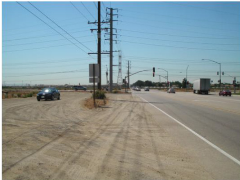
Northern boundary of project site from NE corner of project site looking west along Riverside Drive
