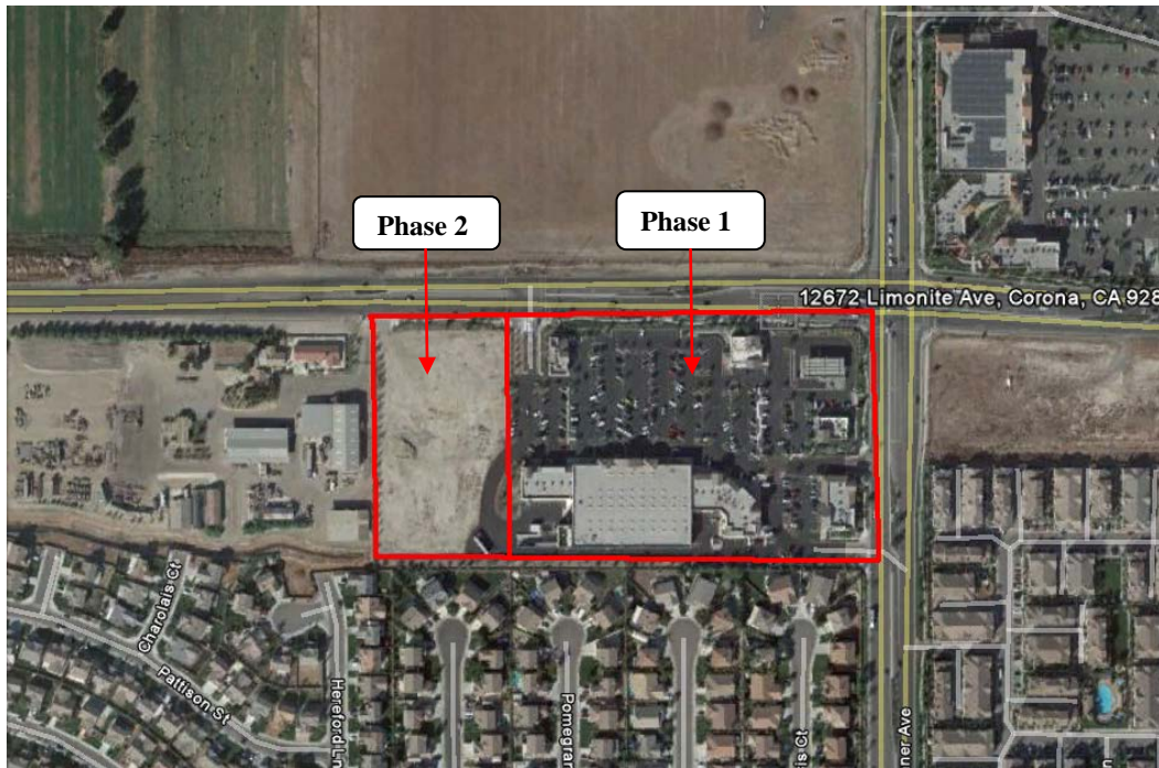
Figure 1: Aerial Photograph of Project Site (Taken Before Completion of Phase 2 Buildings)
