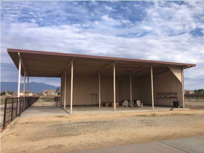
Photograph 9: Open-side shed facing north.
