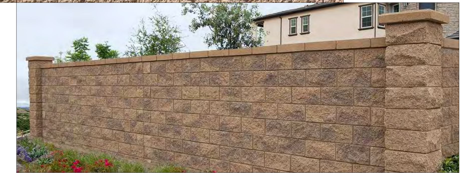
Split face block wall & pilaster
