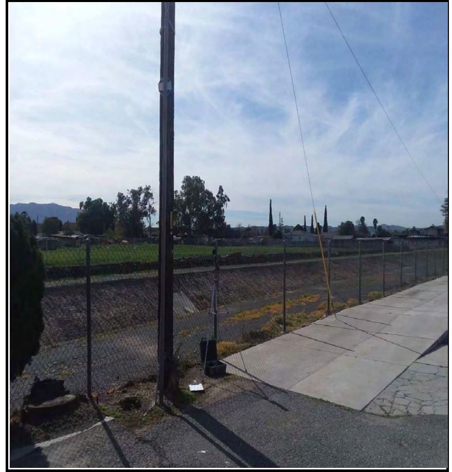
STNM5 looking SW across drainage channel towards northern edge of site ( green field on other side of drainage channel ).
