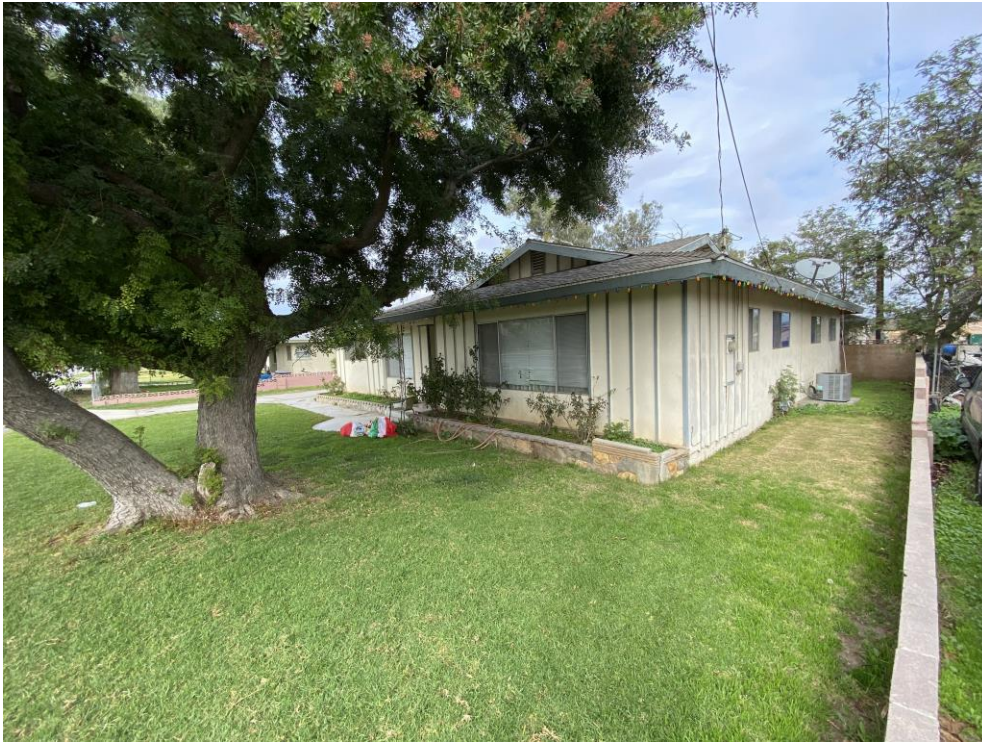
Photo 2: Overview of southeast and east elevations of the residence (View NW)
