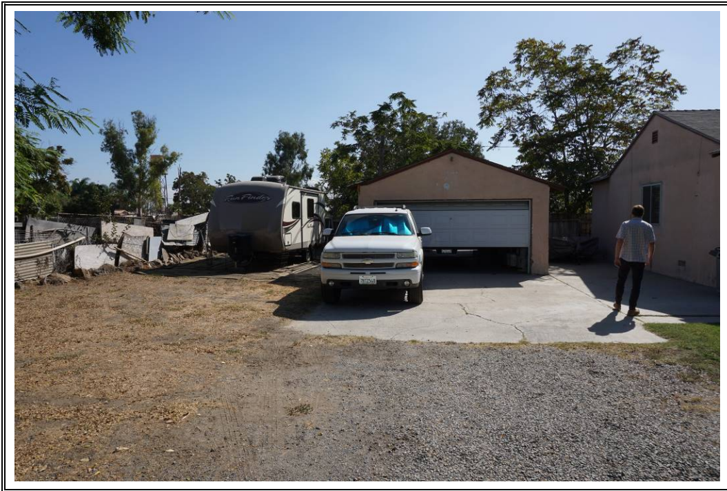
Photograph Number 9: View of detached garage (14557 Chandler Street), facing east.
