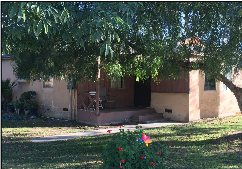
Plate 10: View of the primary (south) façade of the 14555 Chandler Street building.
