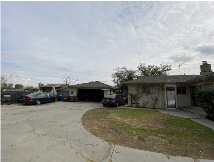
Photo 10: Detached garage behind the residence at 14587 Chandler Street (View E)
