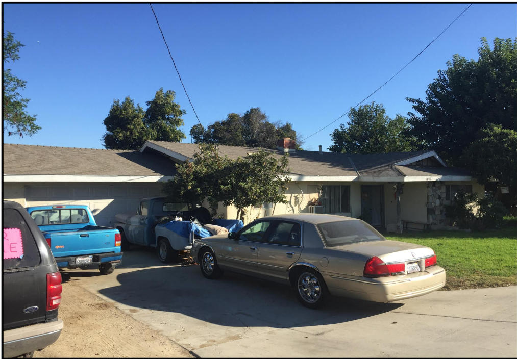
Plate 8: View of the primary (south) façade of the 14577 Chandler Street building.
