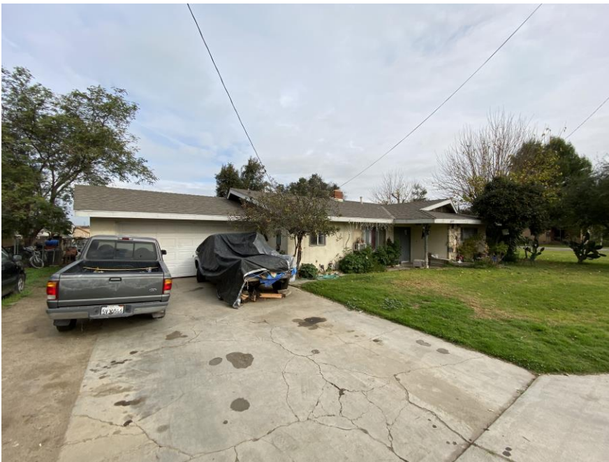
Photo 8: Attached garage at 14566 Chandler Street (View NE)
