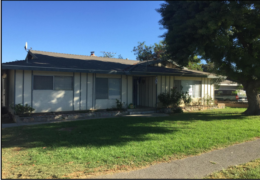
Plate 7: View of the primary (south) façade of the 14581 Chandler Street building.
