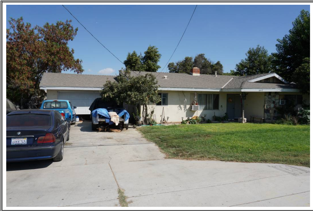
Photograph Number 11: View of subject property dwelling (14577 Chandler Street), facing north.
