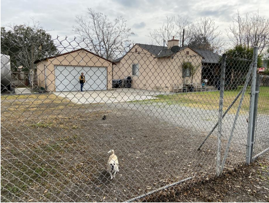
Photo 3: Historic-period residence at 14557 Chandler Street and detached garage (View SE)
