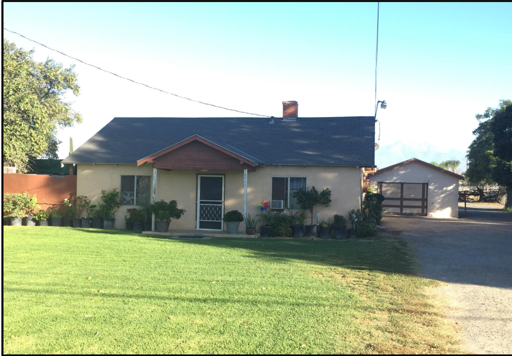
Plate 9: View of the primary (south) façade of the 14565 Chandler Street building.
