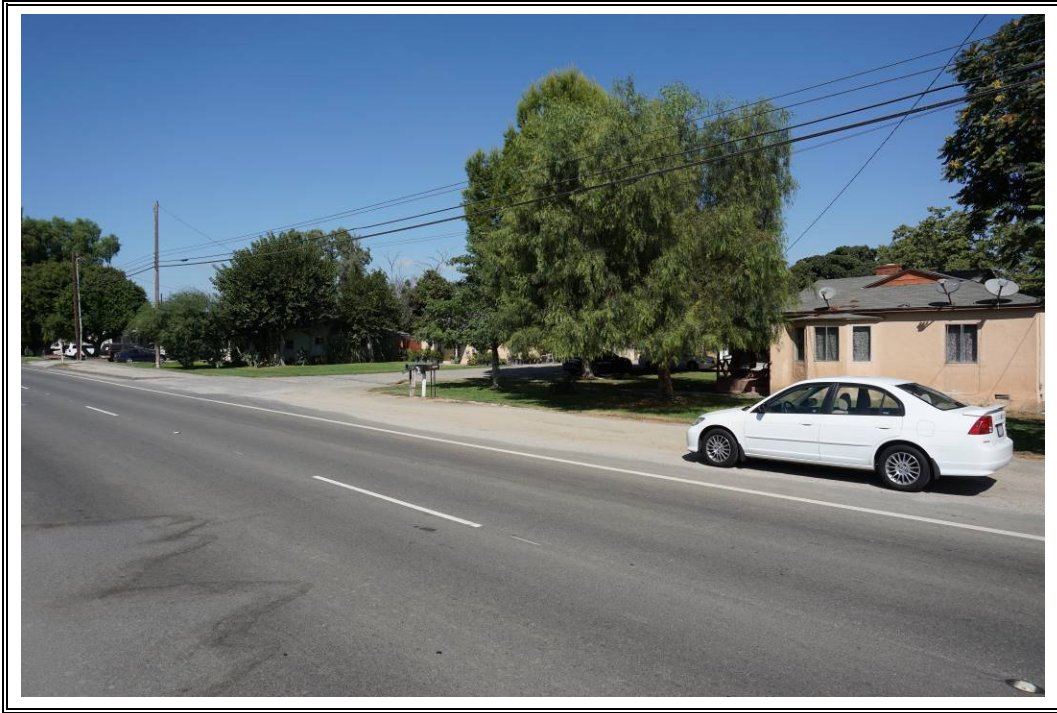
Photograph Number 1: View of south side of subject property along Chandler Street, facing northwest.
