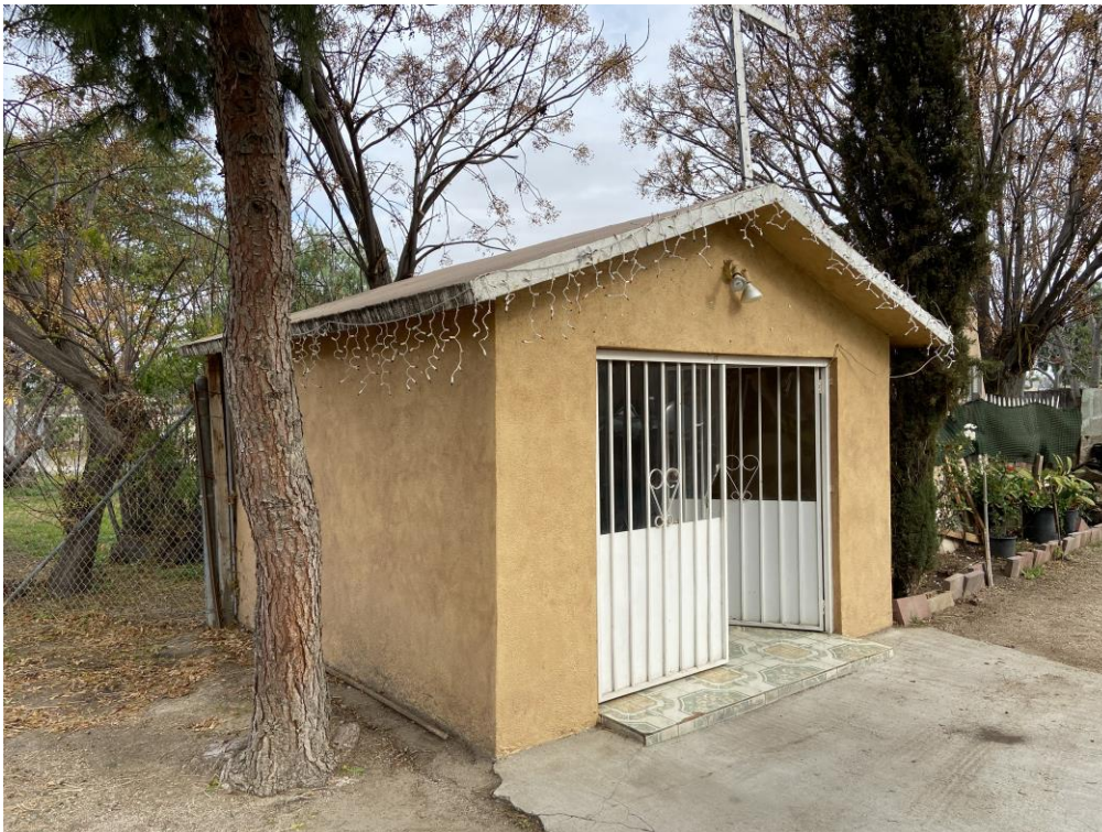
Photo 5: Overview, ancillary structure associated with Building 2 (View NE)
