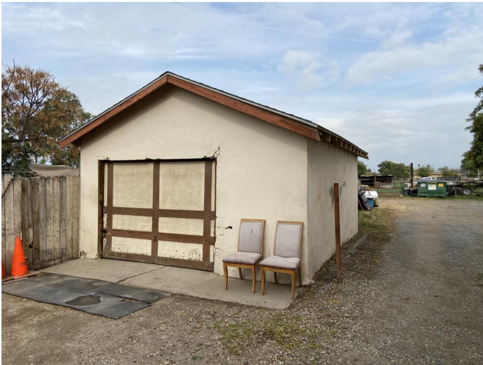
Photo 2: Overview, detached wood frame garage belonging to Building 1 (View NW)
