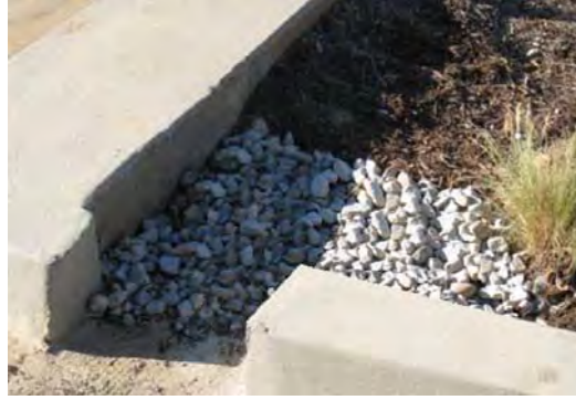
Figure 2: Curb Cut located in a Bioretention Facility
