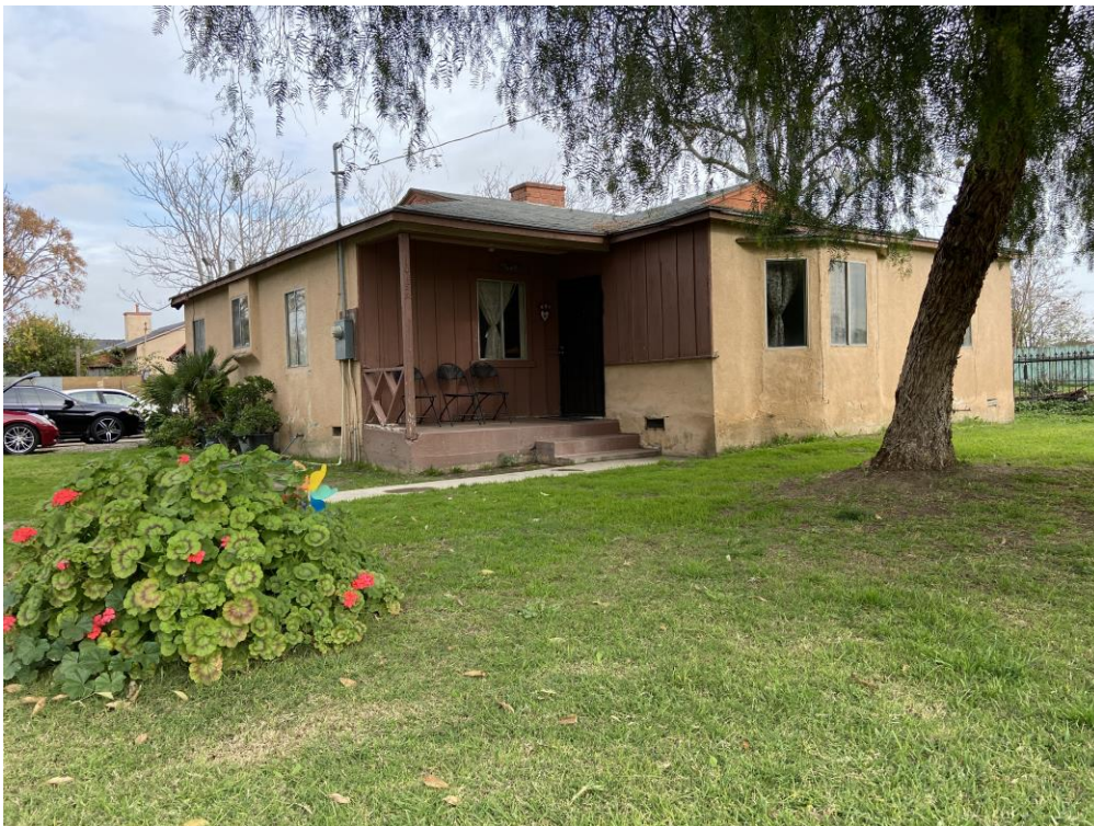
Photo 3: Overview, Building 2 built in 1950 (View NE)
