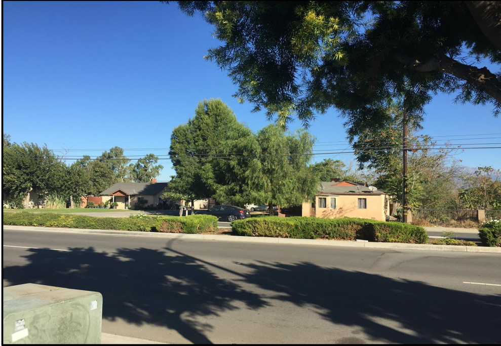
Plate 11: Overview of the 14565 Chandler Street (left) and 14555 Chandler Street (right) buildings, facing north.
