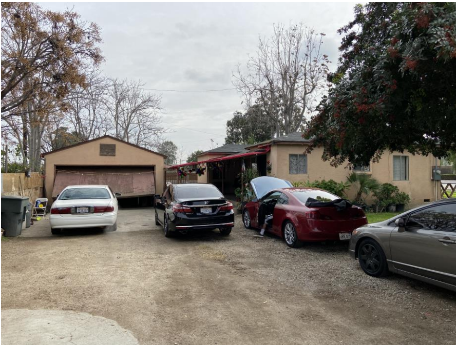
Photo 2: West elevation of 14555 Chandler Street and detached garage (View E)
