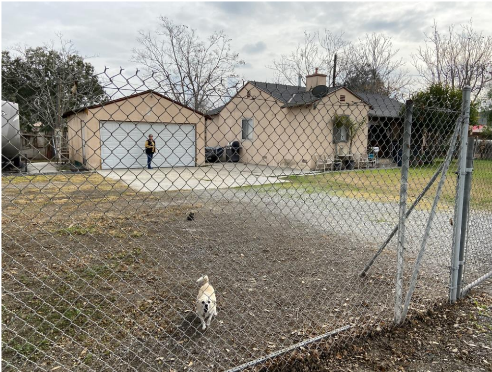
Photo 6: Overview, Building 3 with detached garage (View SE)
