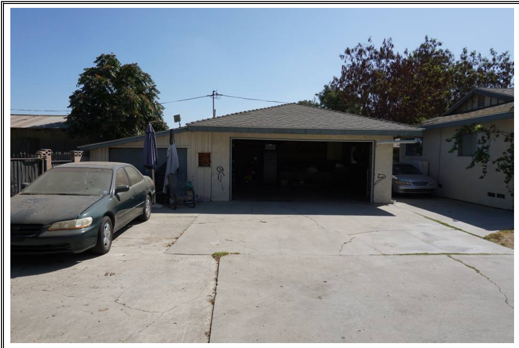
Photograph Number 15: View of subject property detached garage (14587 Chandler Street).
