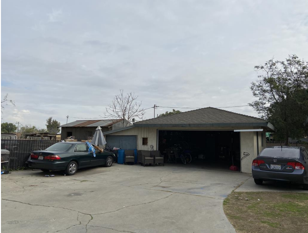
Photo 4: Overview of the two-carport detached garage (View E)
