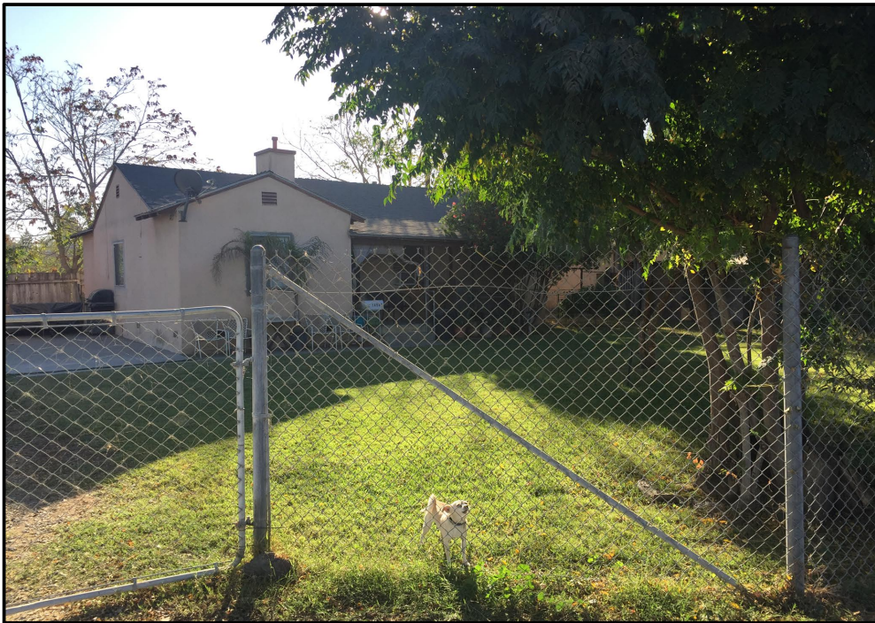
Plate 12: View of the primary (west) façade of the 14557 Chandler Street building.
