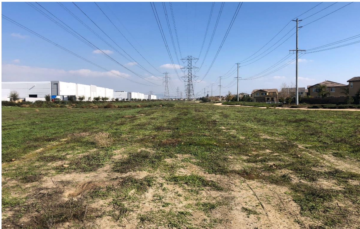
Photograph 8. View from eastern bank of Cucamonga Creek Channel. View to the east.
