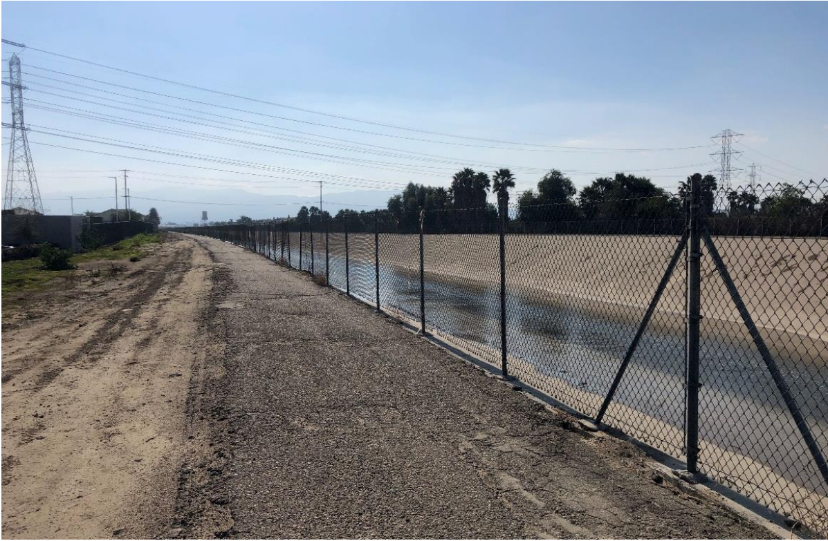
Photograph 2. View of Cucamonga Creek Channel along path west of Parker House warehouse store facing south.
