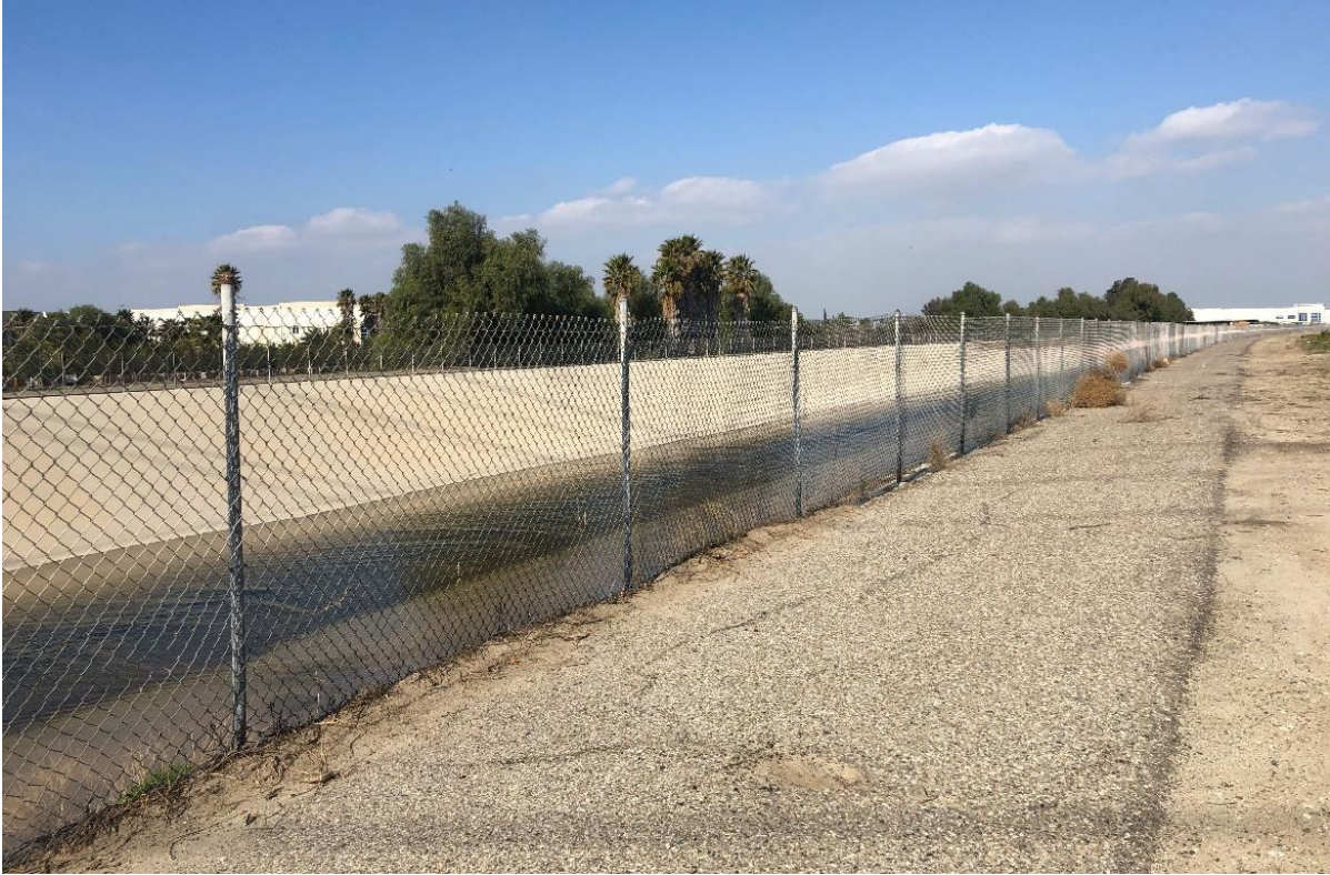
Photograph 1. View of Cucamonga Creek Channel along path west of Symphony Court facing north.
