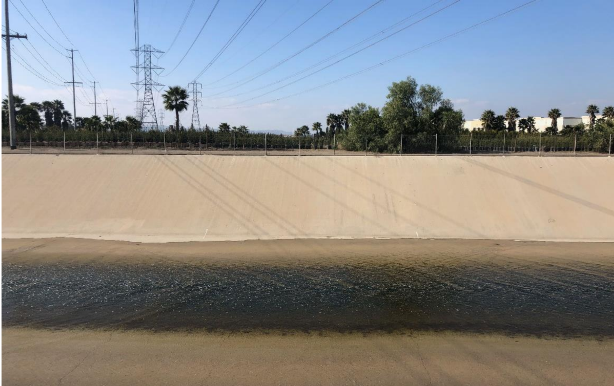
Photograph 3. View across CCC, facing west.
