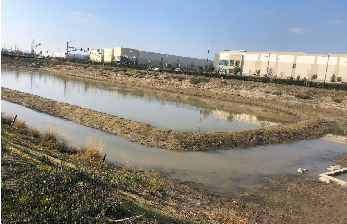
Photograph 7. View of isolated basin created within the industrial area on the west side of the CCC.
