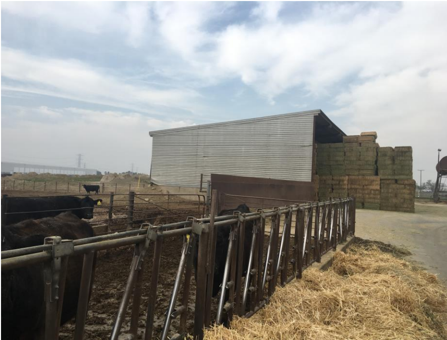
Photo 5: Commodity Barn (W)
