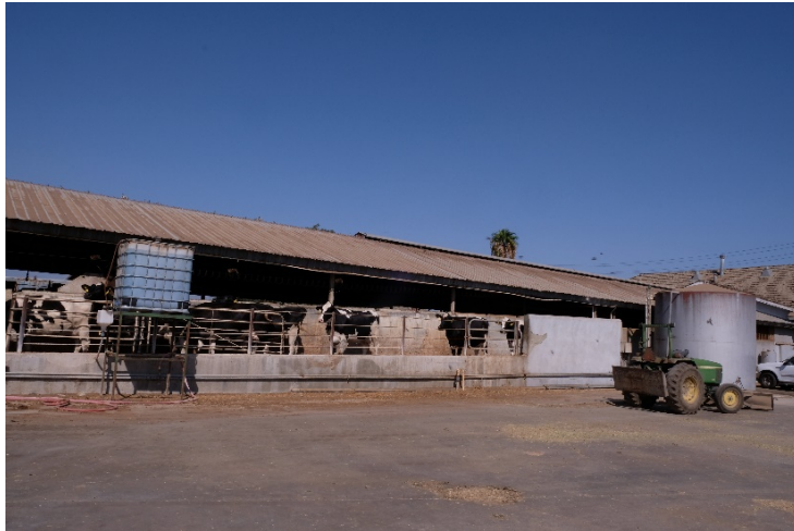
Photograph 3. View north from within site
