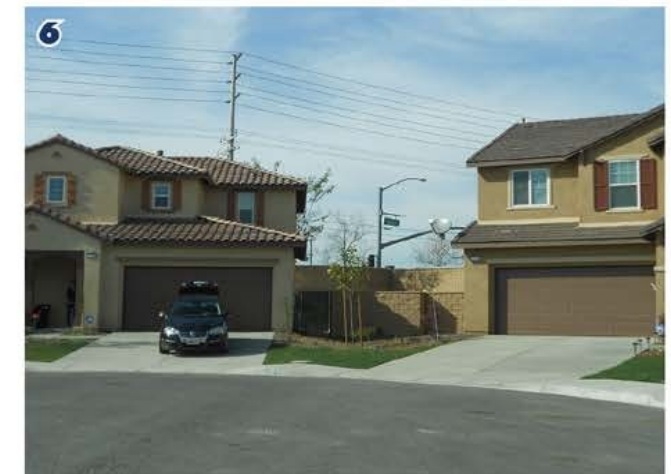
A sound wall behind residential uses reduces noise impacts from traffic along Bellegrave Avenue
