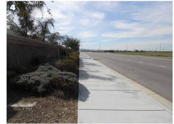
Sound wall, landscaping and sidewalks buffer a residential neighborhood from Bellegrave Avenue
