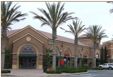
Examples of commercial buildings with appropriate levels of building form and articulation through variations in roof heights, changes in texture, materials, and color, corner emphasis, and building off-sets.
