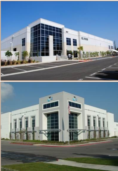
Examples of an appropriate corner treatments as well as features such as changes in colors and scoring that articulate the body of the building.
