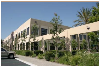
Examples of appropriately articulated buildings including the use of a building cap (top and middle), a building designed without a cap (bottom), and building bases achieved with changes in color and materials (top and middle).
