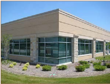
Example of the complementary use of color and material changes to highlight a building's articulation and to blend with the overall architectural expression of the structure.
