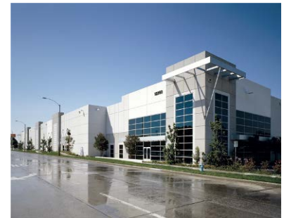
Example of building treatments that help control the mass of industrial buildings, including use of vertical elements, building off-sets, tower elements, and varied roof-lines.
